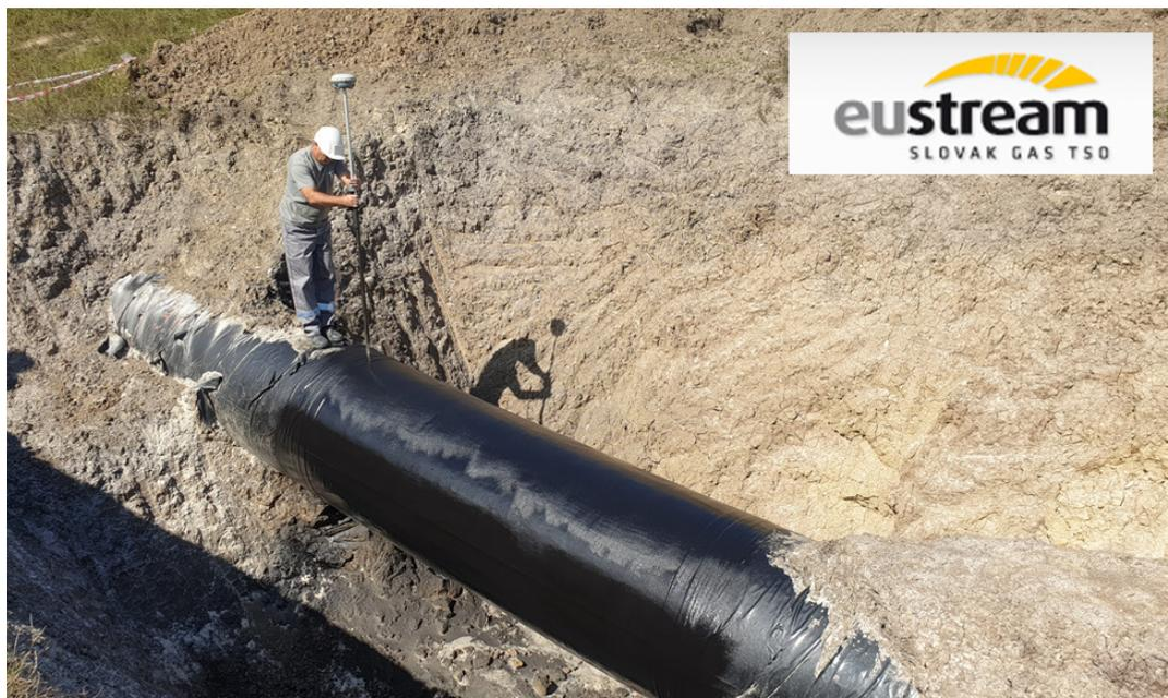
*Eustream's field operator measuring the location of a gas pipeline with a GNSS receiver. Credits: Eustream*
